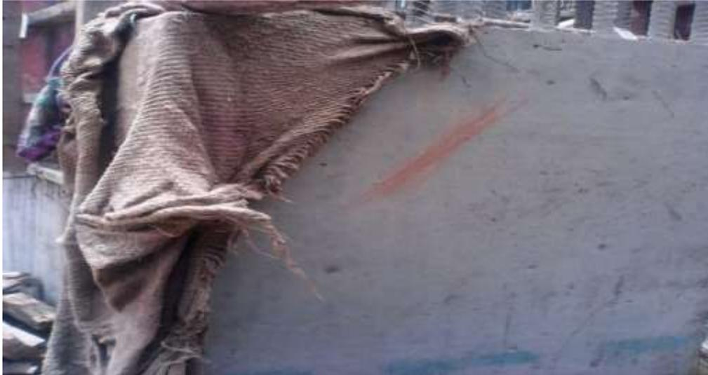
Curing should be started just after the surfaces begin to dry. Normally 7 to 15 days curing is adequate.
